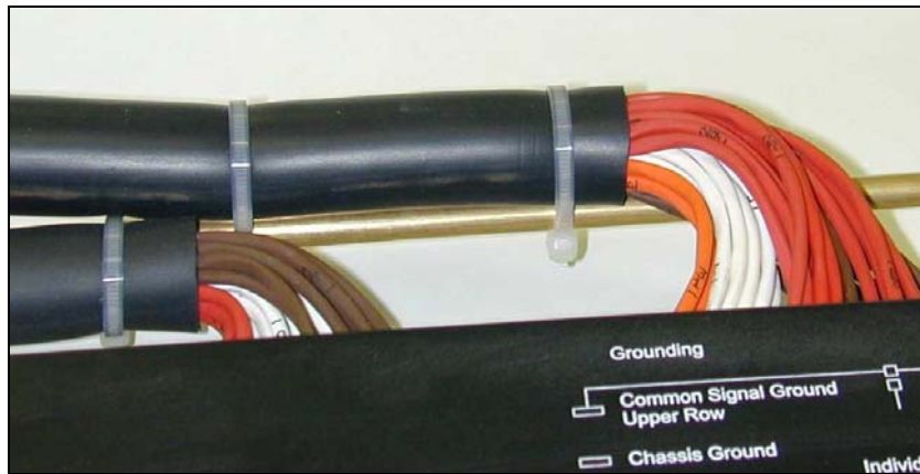
Cable Retention Bar
